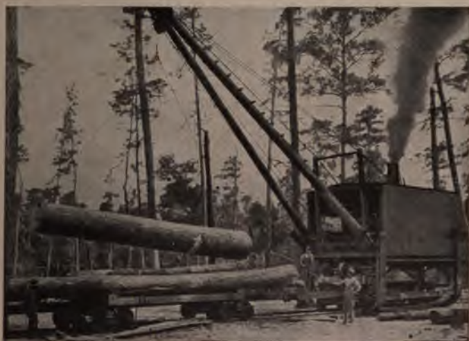
FIG. 95. — A McGiffert Log Loader.
